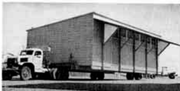
Portable Classroom Being Moved
